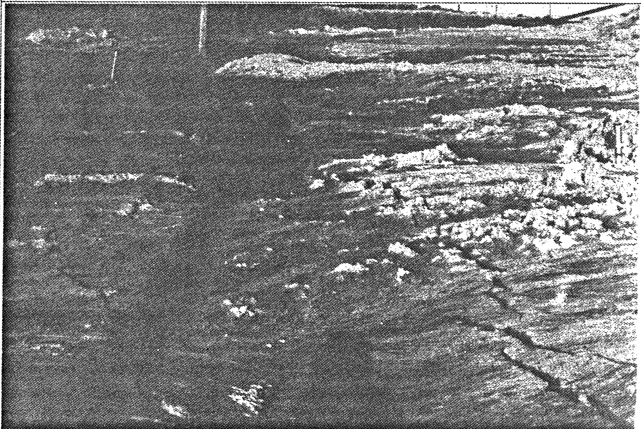
Figure 13 -Cracking on Berm
