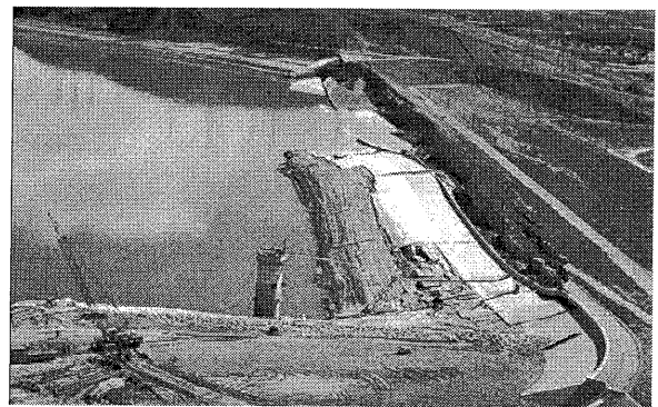
Fig. 1. Failure of the lower San Fernando dam.
